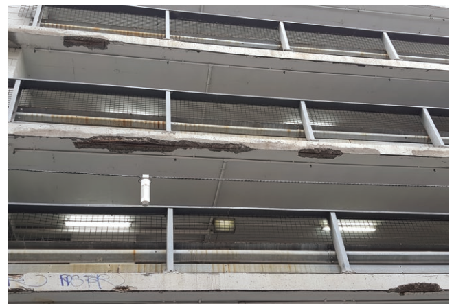
A multi-storey car park suffering from spalled concrete due to corrosion of the rebar
