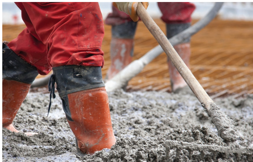
Racking concrete
