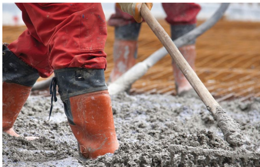
Racking concrete
